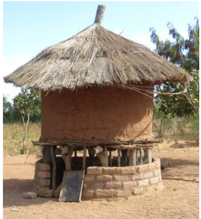
Figure 9: A goat nursery constructed below grain storage, offering predator protection.
